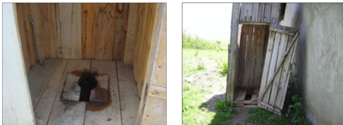
Figure 17 “The common household unimproved pit latrine”
