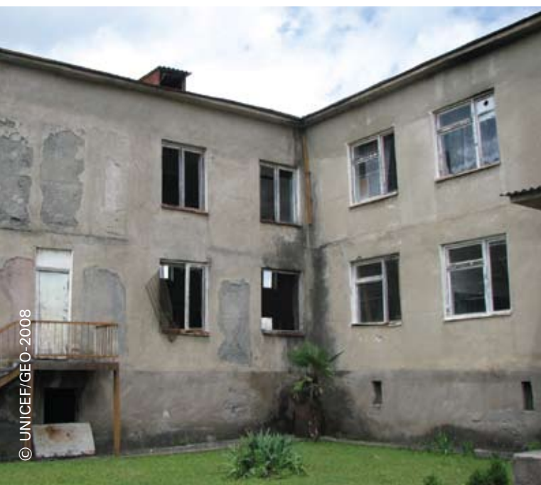
School in Kindigh before and after rehabilitation
