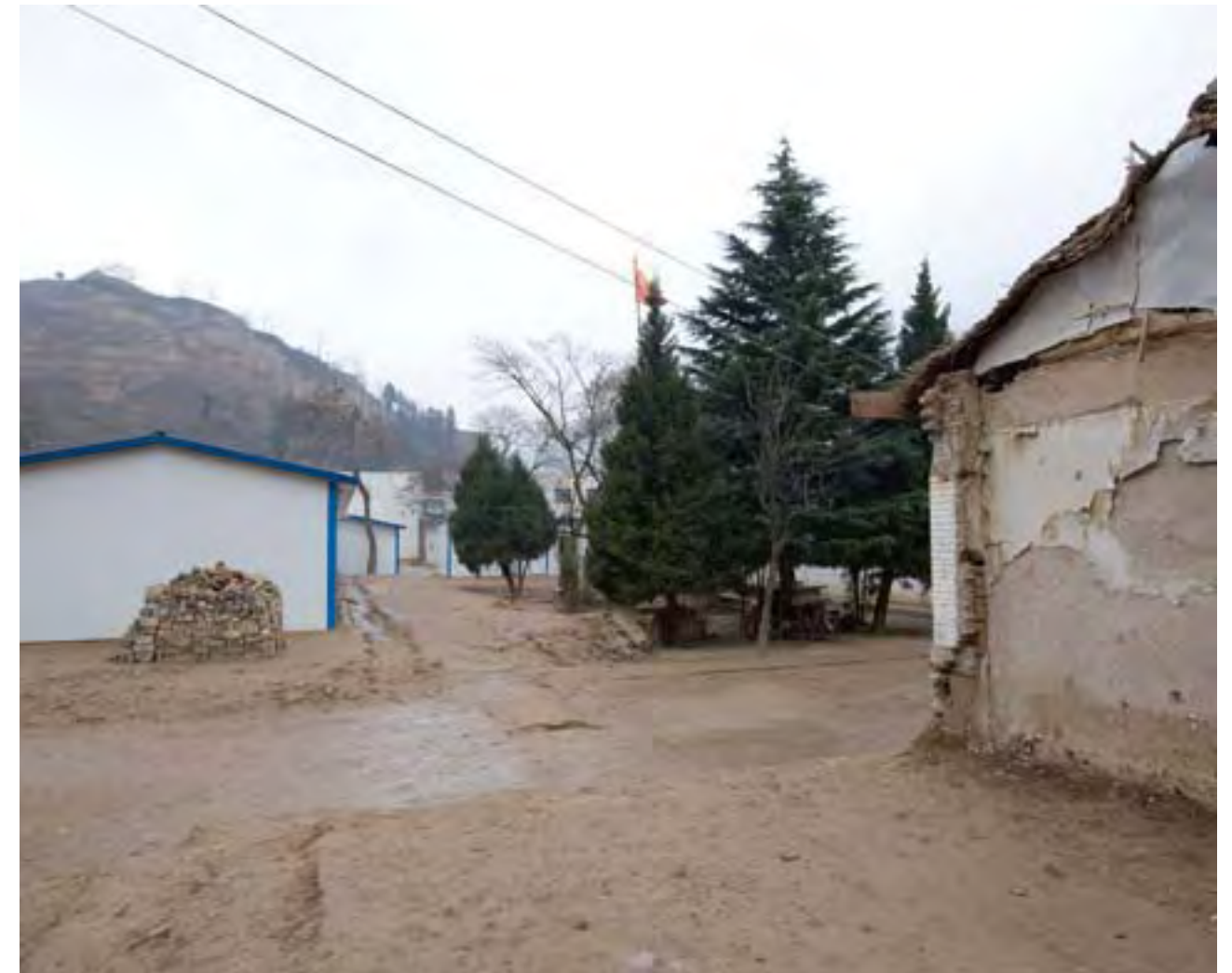
Prefabricated classrooms help students whose schools were severely damaged in Xihe County, Gansu Province return to a safe learning environment.
