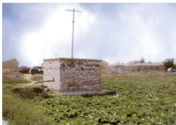
Figure 9: Pumping station of an arsenic-safe piped water supply system, Inner Mongolia autonomous region, China
