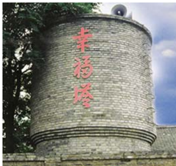
Figure 10: A water tower of an arsenic-safe piped water supply, Shanxi province, China
