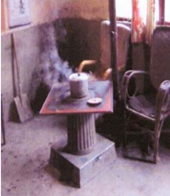
Figure 12: An improved stove with chimney has replaced the conventional open stove in a rural household, Guizhou province, China
