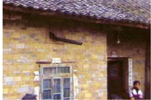
Figure 13: The chimney of the improved stove vents away the arsenic-contaminated smoke in the house, Guizhou province, China
