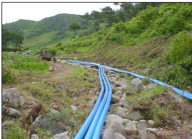
Gravity water system under development in Kosan County, Kangwon Province
